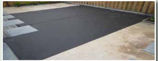
Step 2 – Apply Membrane/Pressure Distribution Cloth
