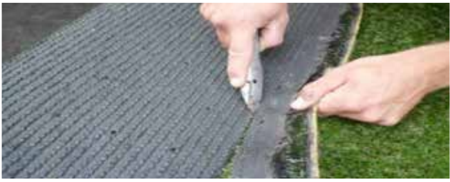
Step 3 – Cut Artificial Grass To Size
