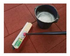
To achieve improved stability we recommend adhering the first and last row of the layout using Castle XP - 2435 PU Adhesive where no edge restraint exists.
