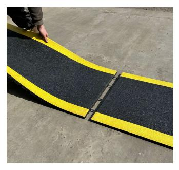
To achieve improved stability we recommend adhering the tiles at the edges using Castle XP 2435 PU Adhesive. Castle XP 2435 adhesive is available in 1 litre bottles with nozzle for application. Adhesive should be applied to the back of the tile taking care not to block the drainage channels as shown in the image below. Applying the adhesive to the back of the tile is important as it allows gravity to pull the adhesive down into contact with the substrate when curing.
