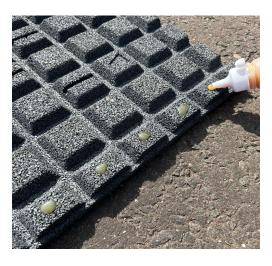
Adhesive should be allowed 24hrs to cure before trafficking. When curing the adhesive will absorb moisture from the atmosphere and expand. The adhesive can be used in damp conditions but this will increase expansion.
