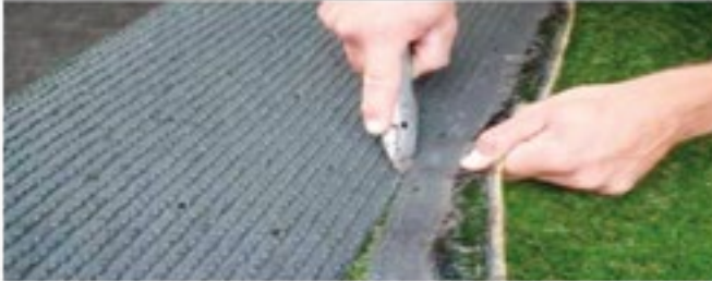
Step 3 – Cut Artificial Grass To Size
