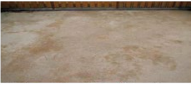
Step 1 – Apply Foundation For Artificial Grass
