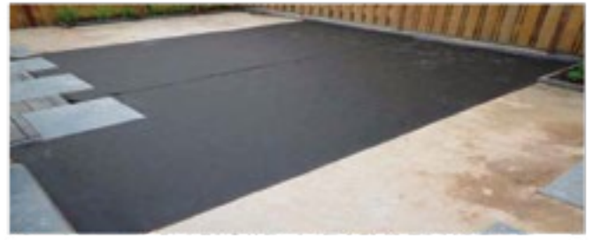
Step 2 – Apply Membrane/Pressure Distribution Cloth
